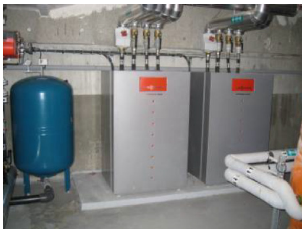
FIGURE 12 : POMPES A CHALEURS VISSMAN VITOCAL 300
