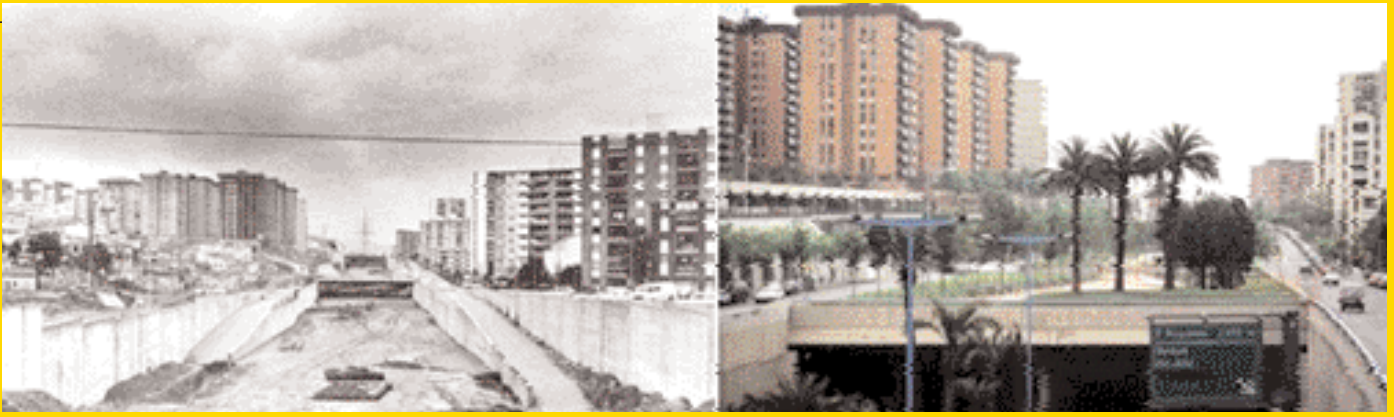
The district of La Ronda de Dalt before and after
