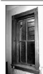
Following the relatively simple repairs, the window is weather-tight, like new in appearance, and capable for many years to come. Photo: NPS files.
