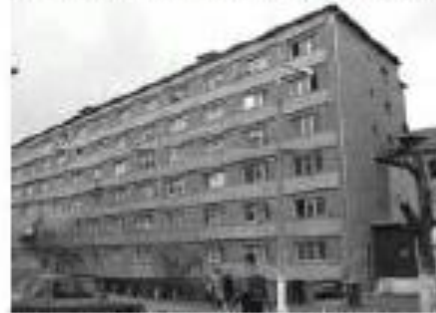
Fig. 1 Main facade of the hostel 20C
