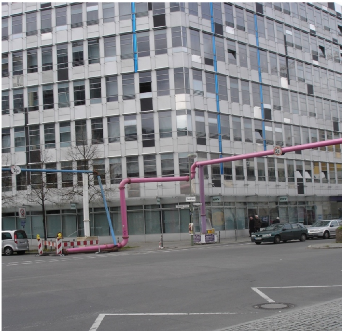
Photo: Berlin-Mitte, travaux et tuyaux, 2008 (C. Huchard-Flory).
