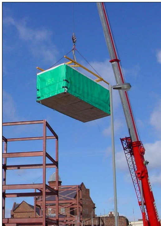
Picture of modular construction of a UNITE property in Bristol
